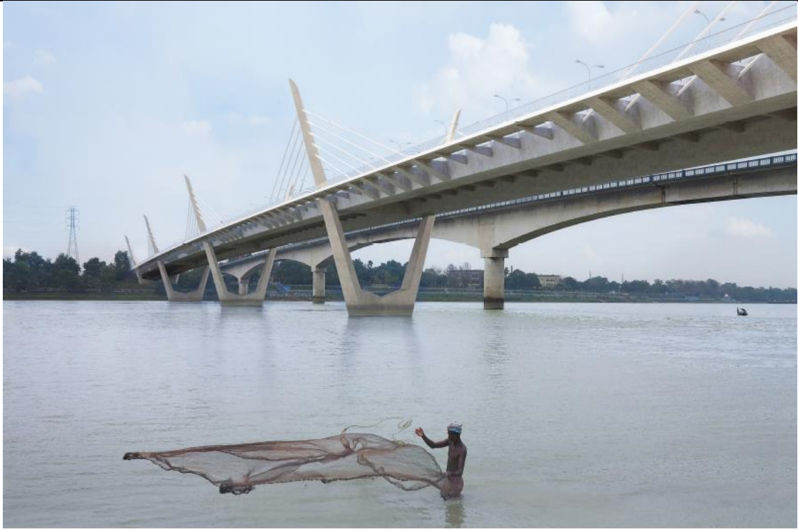
Design Support during implementation stage: 6-lane extra dosed bridge over Ganga River Near Kalyani adjacent to existing Iswar Gupta Setu, West Bengal
