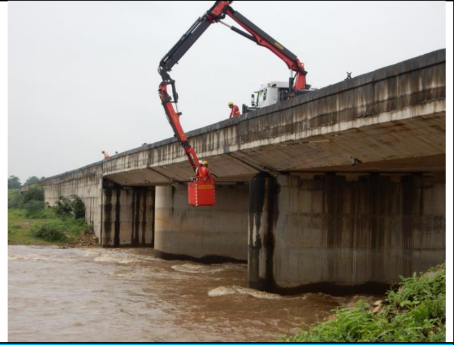
Inventory & Condition Survey of Bridges using Mobile Bridge Inspection Unit (MBIU), Andhra Pradesh
