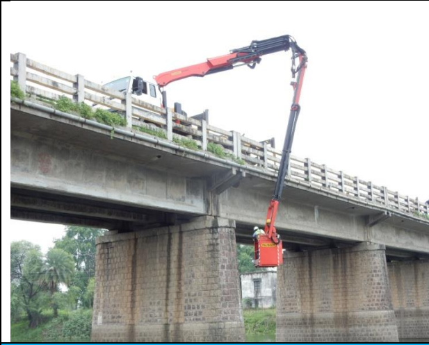
Inventory & Condition Survey of Bridges using Mobile Bridge Inspection Unit (MBIU), Andhra Pradesh
