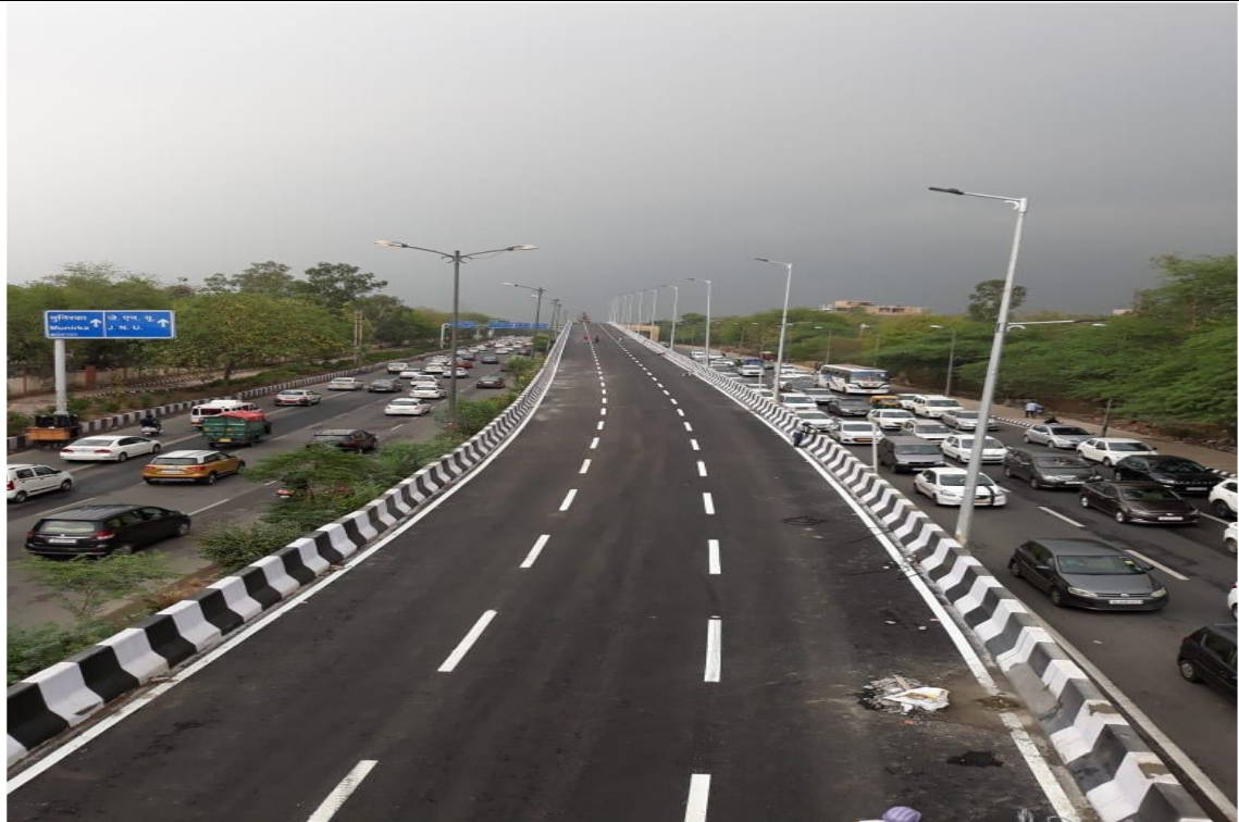
Third Party Inspection & Quality Audit for Rao Tula Ram Elevated Flyover, Delhi
