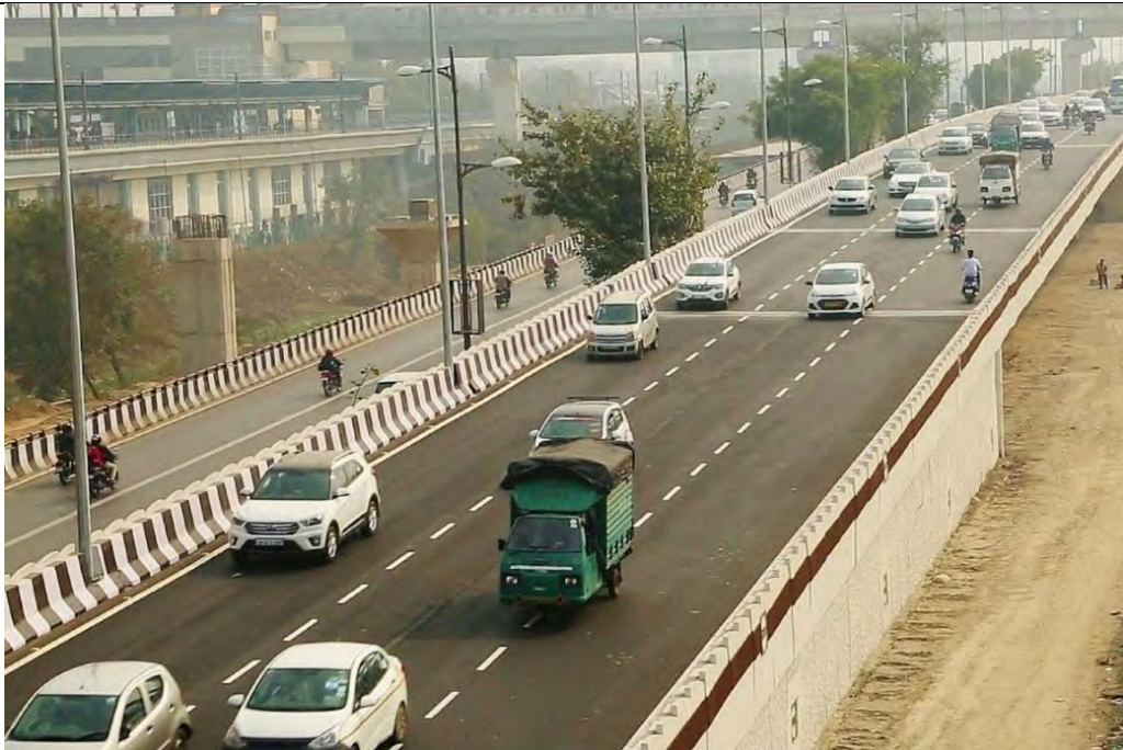
Third Party Inspection & Quality Audit: Completed Elevated Road; Mayur Vihar - Akshardham Section (6-lane), Barapullaha Phase-3, Delhi
