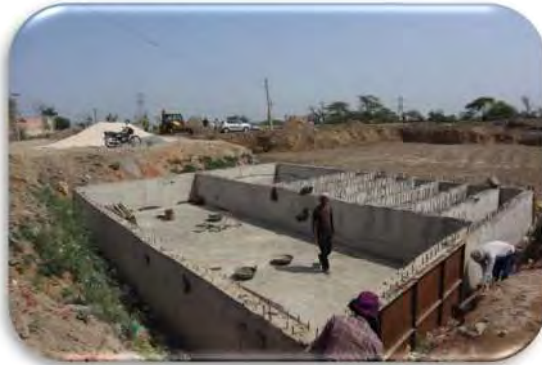
Restoring Jhod in village Budhera, Gurgaon, Haryana
